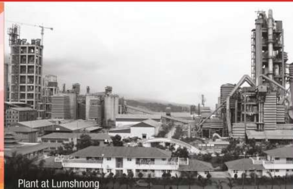
Plant at Lumshnong
